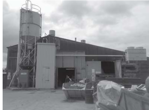
Overall view and with USR protected from the elements.
