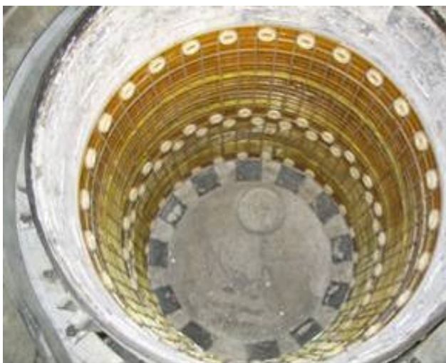
Installation of OCP sensor cable
